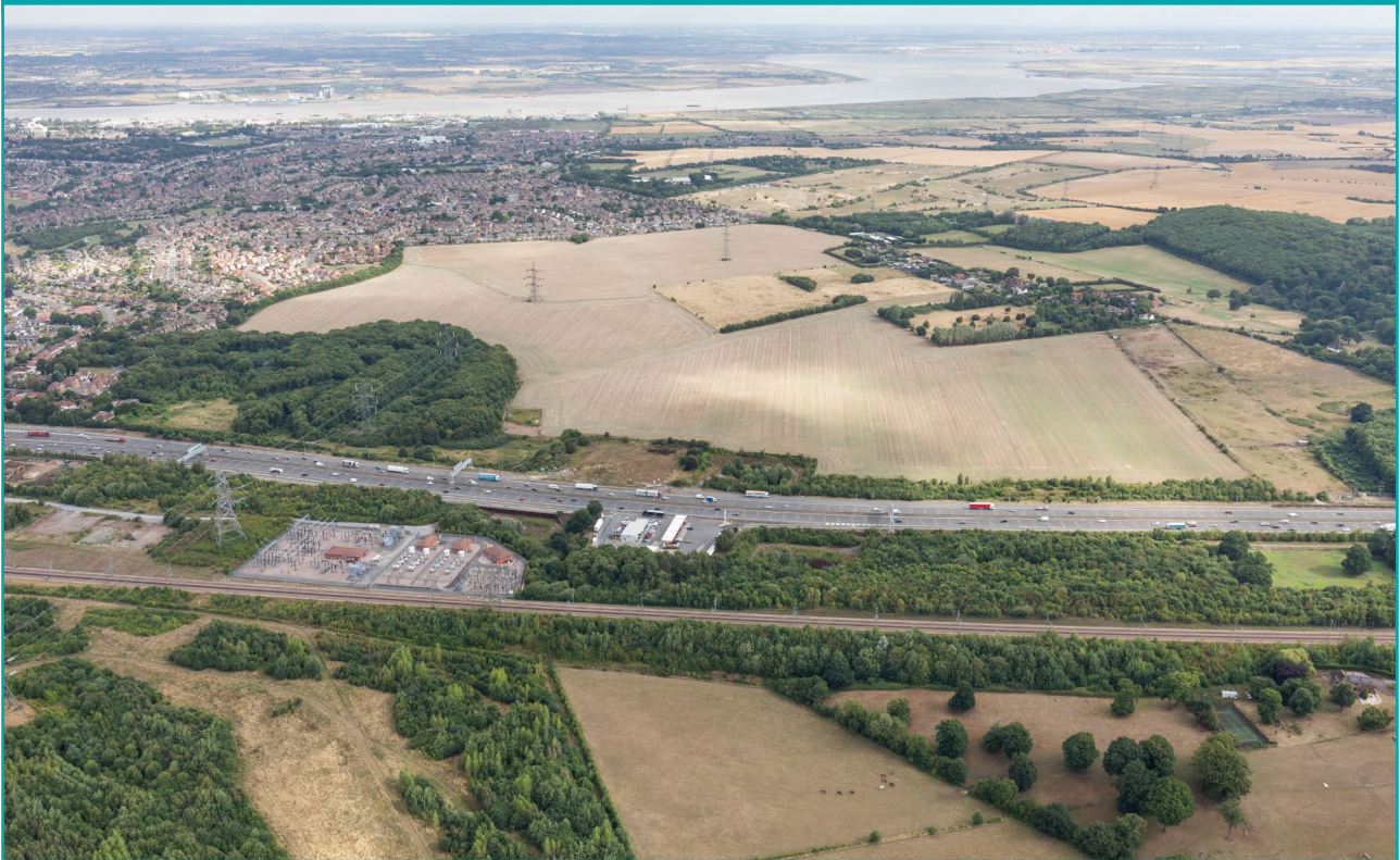
Figure 5-13. Existing A2, looking north
