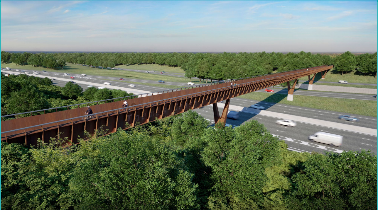
Figure 5-67. Community impacts consultation – proposed walking, cycling and horse riding bridge over the M25 connecting to the Thames Chase Community Forest, looking south-west
