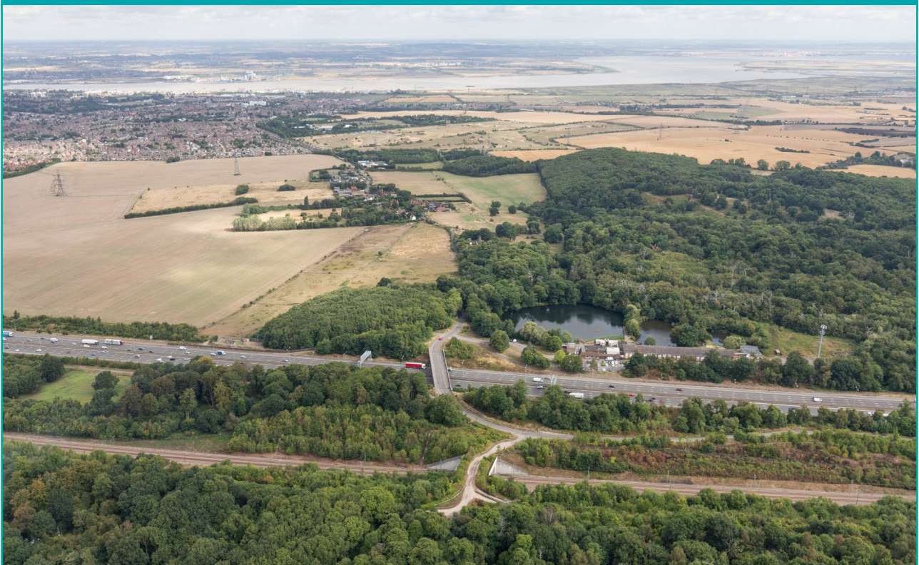
Figure 5-18. Existing Thong Lane and A2, looking north
