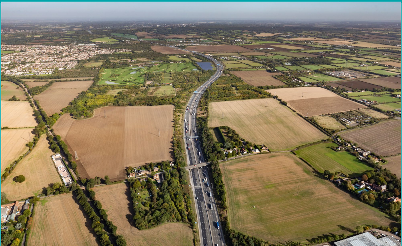
Figure 5-63. Existing M25 and Ockendon Road, looking north
