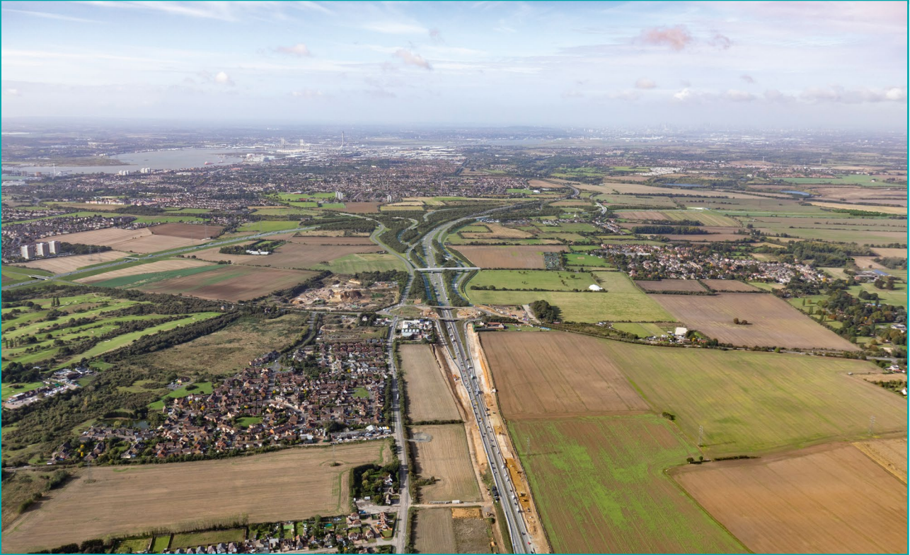
Figure 5-51. Design refinement consultation – proposed view east of A13/Orsett Cock roundabout and A1013 Stanford Road, looking west
