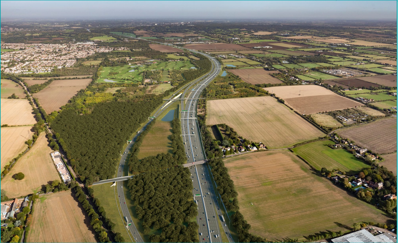
Figure 5-64. Supplementary consultation – proposed LTC/M25 junction, with new Ockendon Road bridge, looking north
