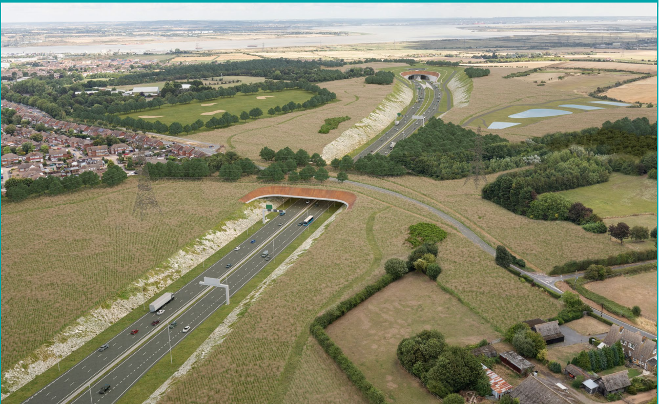
Figure 5-5. Supplementary consultation – proposed Thong Lane green bridge linking Gravesend and Thong and the approach to the southern tunnel entrance, looking north
