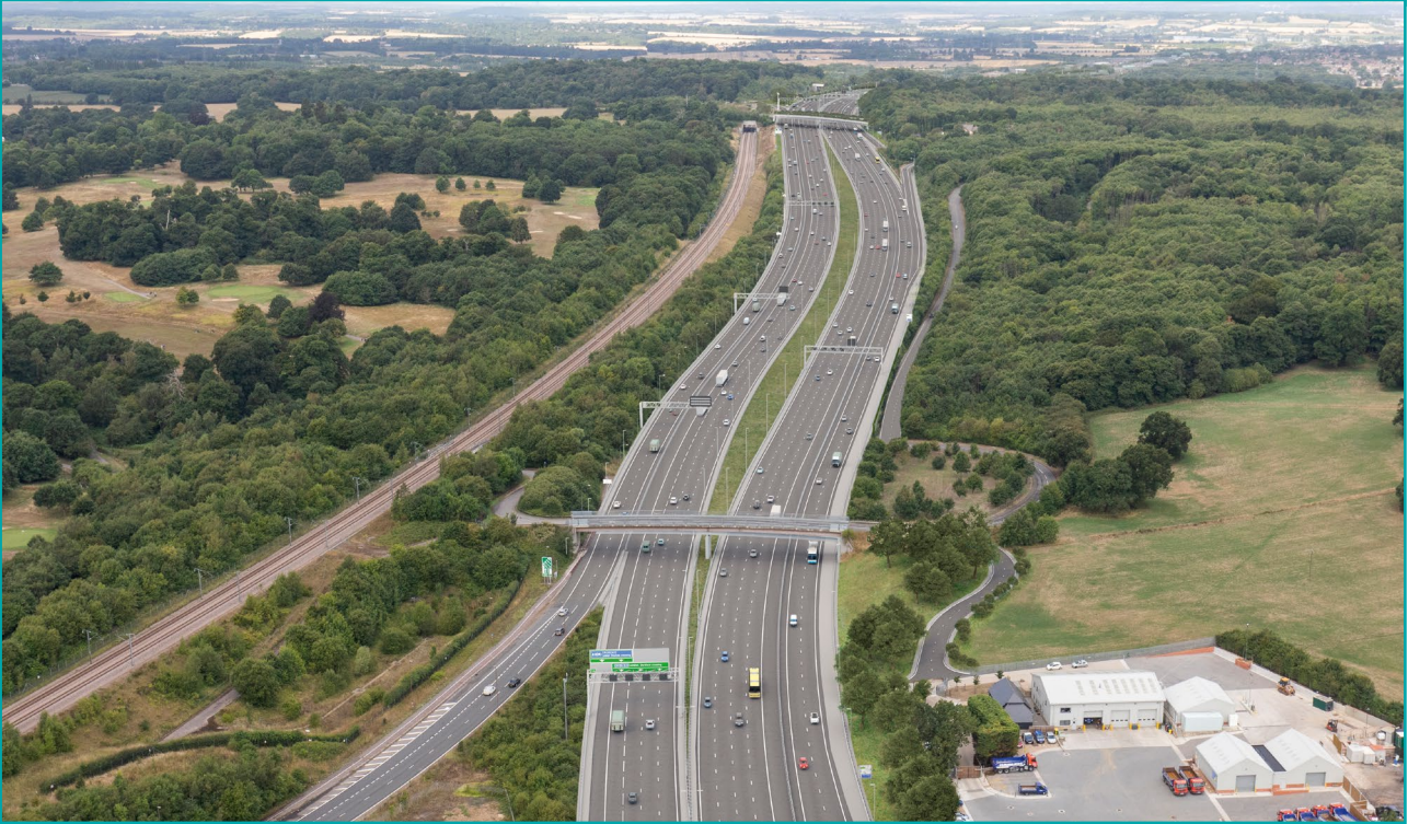
Figure 5-9. Statutory consultation – proposed M2/A2 along the A2 near Park Pale bridge, looking west
