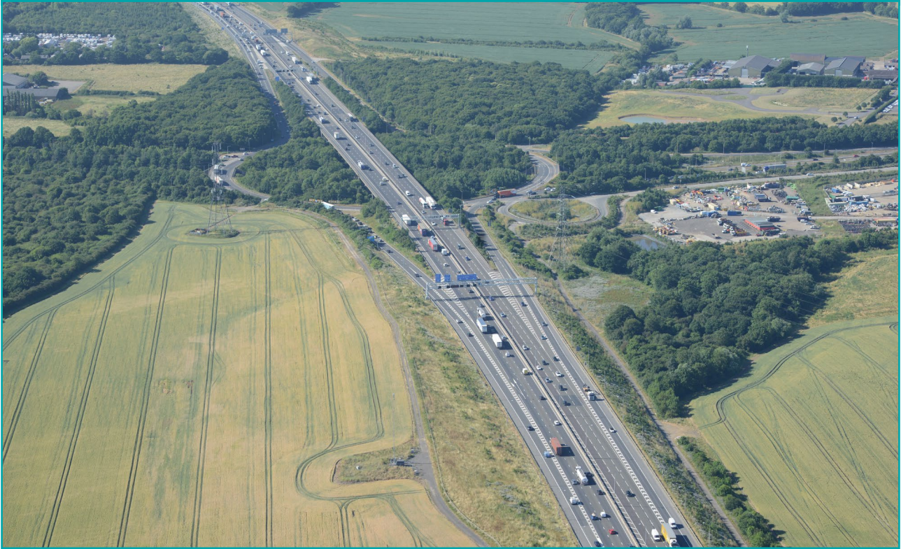
Figure 5-69. Existing view of M25 between junction 29 and 30, looking north
