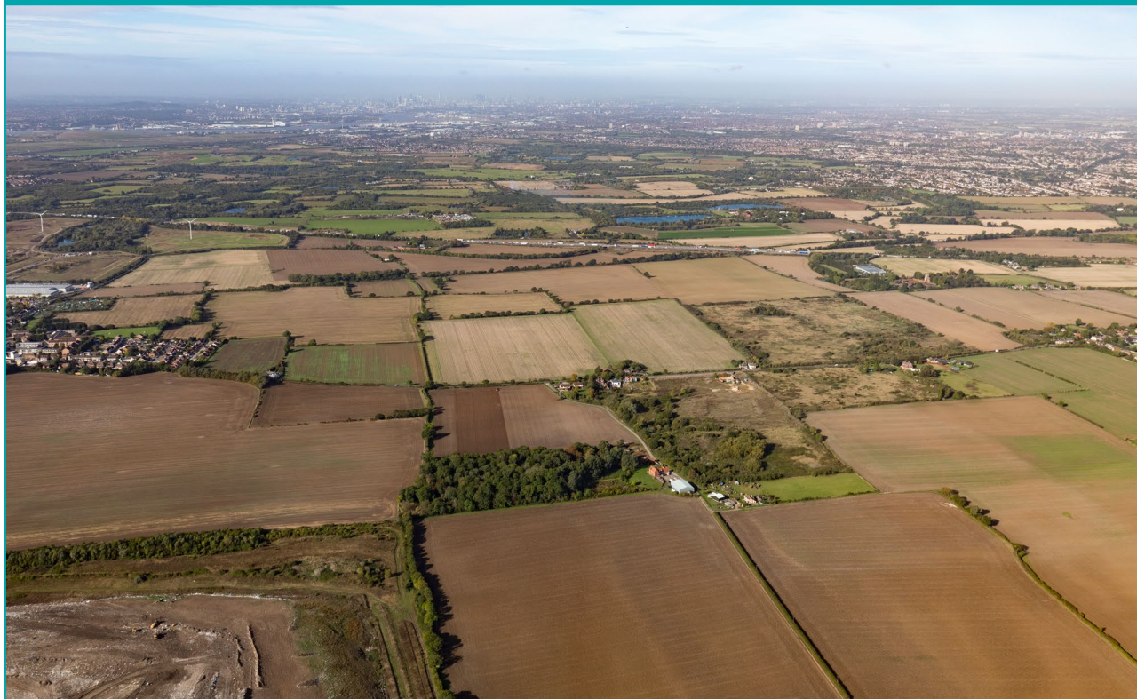
Figure 5-58. Existing North Road, looking west
